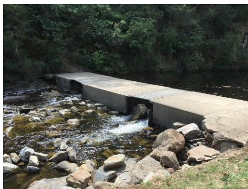
Figure 1 – Snow Creek Weir – existing structure
